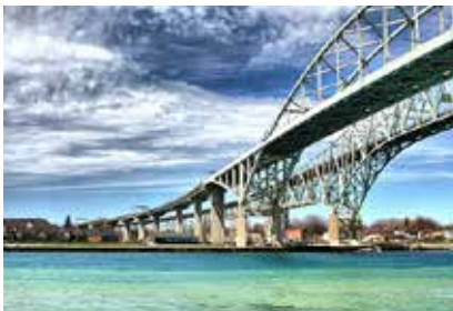
BLUE WATER BRIDGE
